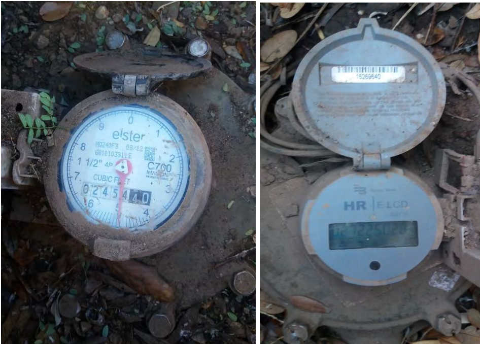
Fig. 4. Analog irrigation meter (left) is read by a person. The new digital irrigation meter (right) is read remotely by the City and we were able to obtain historic irrigation application data from both meters.
