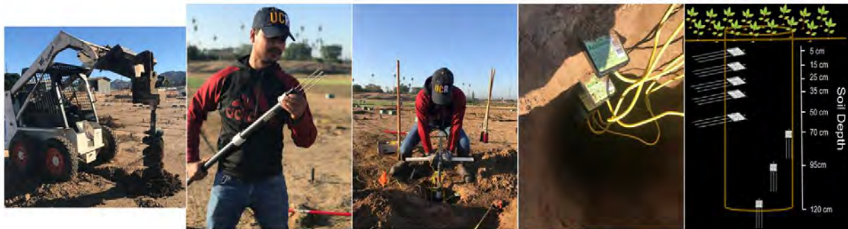
Figure 2. TDR sensors installation steps at different depths.
