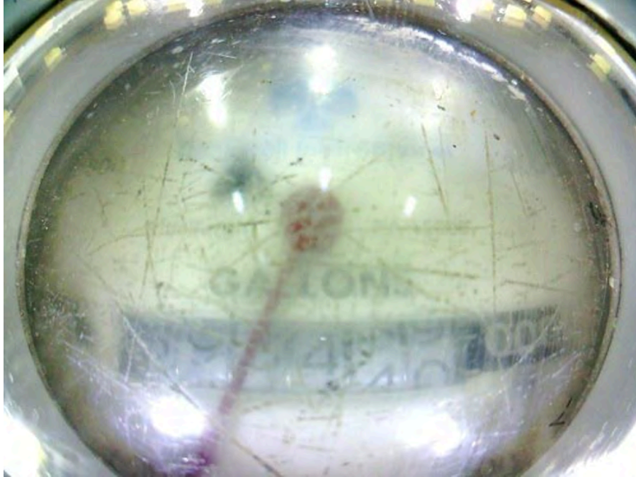
Figure 19 - Damaged register which makes meter reading difficult and prone to misreads.
