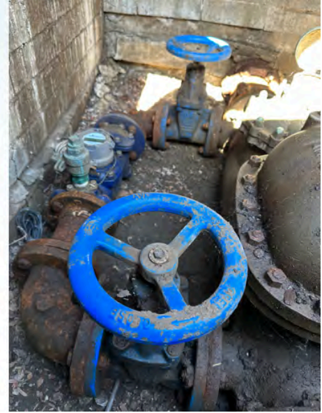
Figure 21 - Damaged register & incorrect meter configuration
