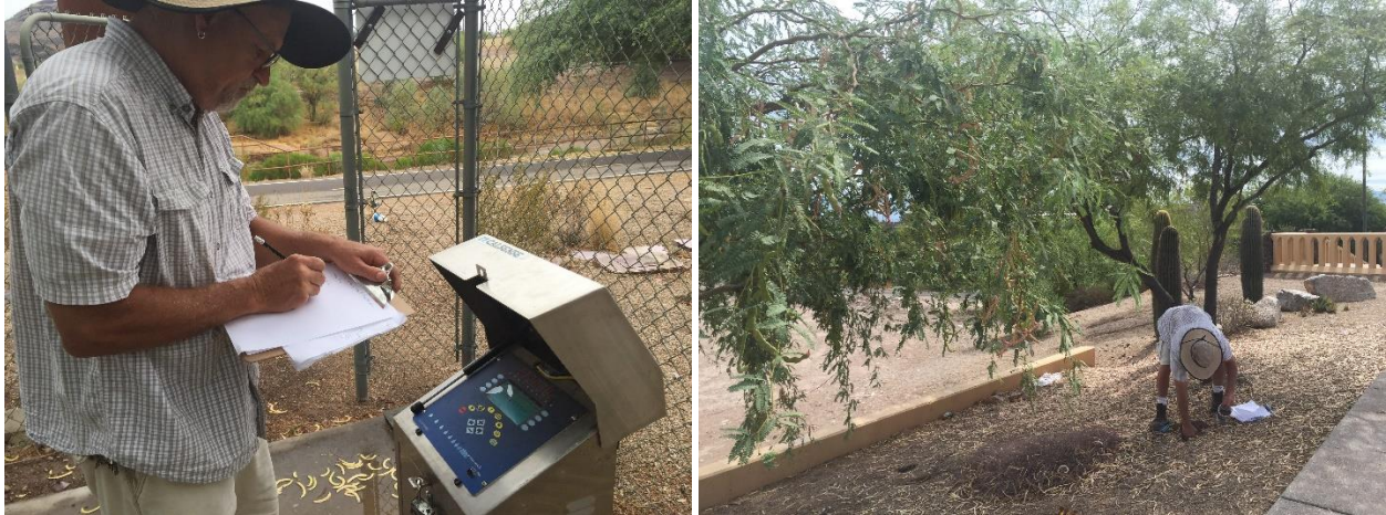
Jeffrey Gilbert audits the CALSENSE irrigation controller for a right of way landscape (left) and is locating number of emitters per tree (right).
