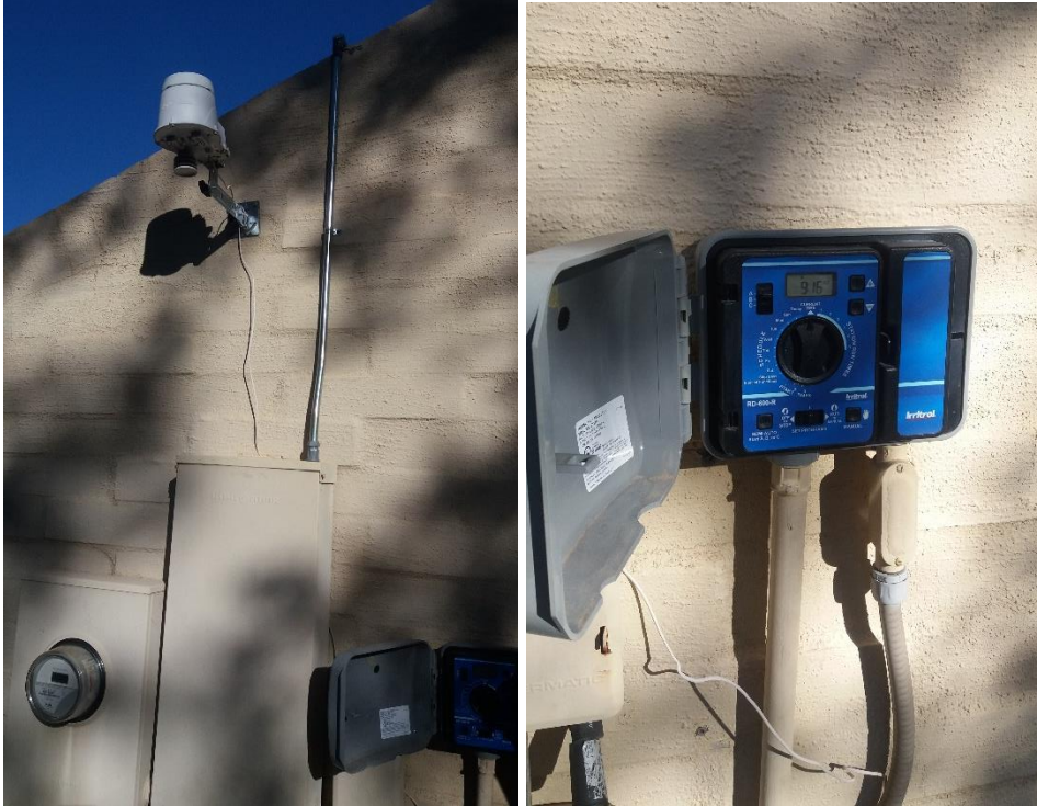
Fig. 3. This property has a Smartcontroller with a weather station, however, the weather station is not hooked up to the controller, thus not providing the required data.
