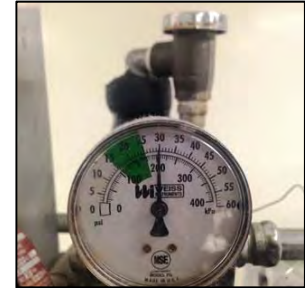
Figure 67: Rinse pressure at 30 psi during operation
