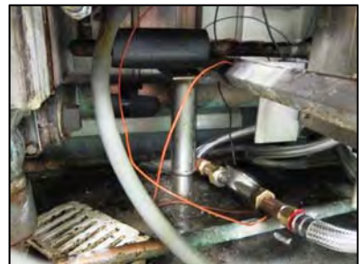
Figure 21: Mechanical meter installation on inlet to booster
