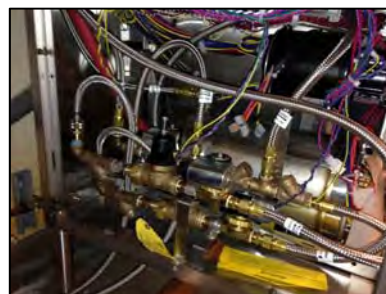
Figure 53: Hobart dishwasher internals
