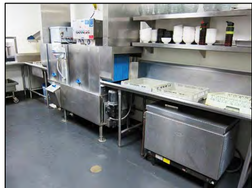
Figure 13: Baadal dishwasher with gas booster
