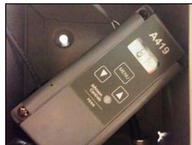
Figure 68: Tempering controls set at 87°F
