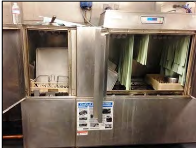
Figure 40: Conveyor jam caused by sheet pan rack loading
