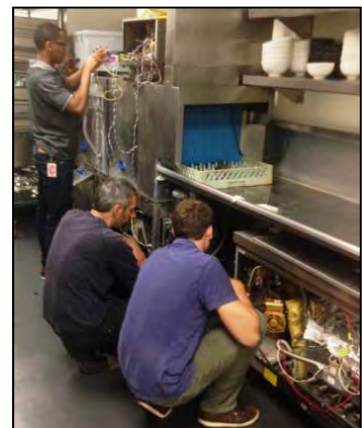
Figure 3: Installing instrumentation on a rack conveyor with booster heater
