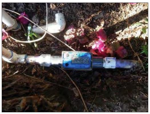
Figure 2. Photo of sub-meters installed at a residential property.
