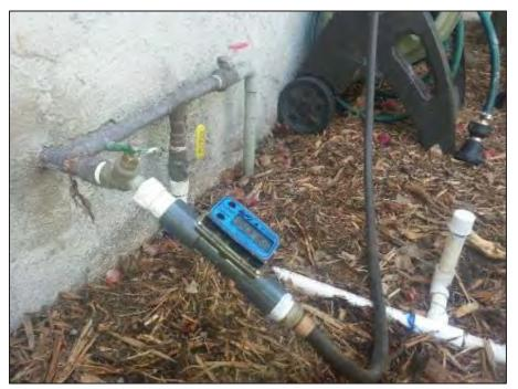
Figure 10. Sub-meter attached to hose for post-implementation watering.
