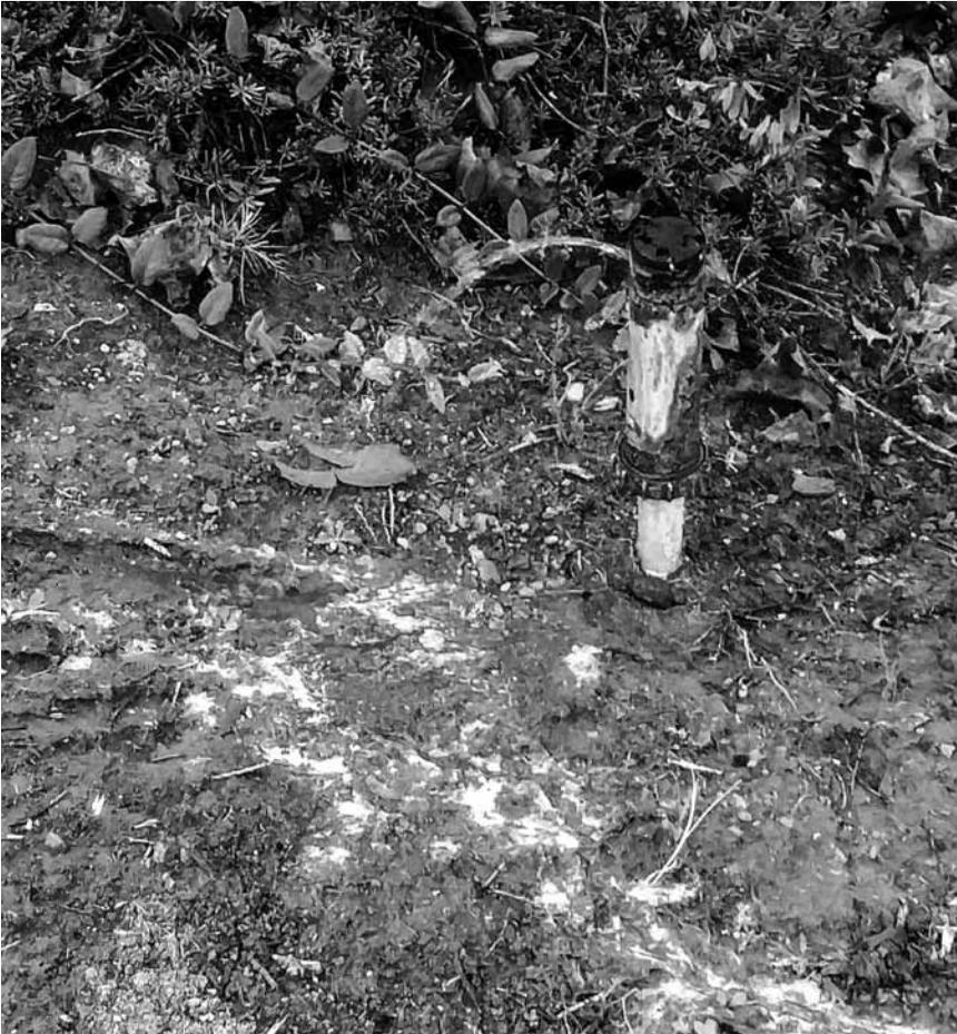
The sprinkler head pictured continues to dribble water long after the valve has been shut off. The ruts in the soil as a result are obvious. The remedies are to install a sprinkler head with a check valve, raise the head, or shore up the slope around the head with large drain rock.
