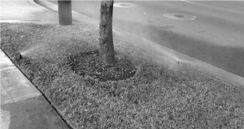
The street and driveway are noticeably wet. The mist produced from these sprinkler heads has been caught by the wind. The water pressure needs to be reduced and/or the heads replaced.
